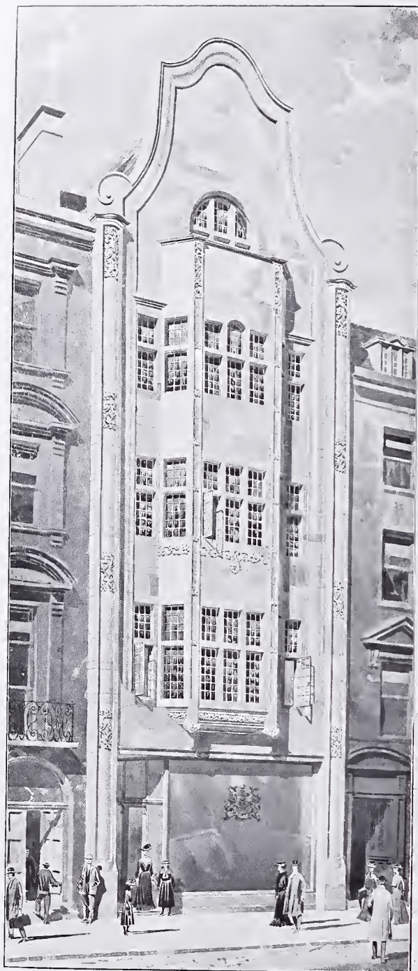
No. 20 Conduit Street, W., TREADWELL AND MARTIN, Architects. Steel Construction; Smith Walker and Co., 11 Tothill Street, Westminster, S.W.
